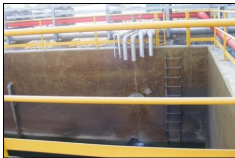
Figure2. Water Sampling at CBD Water Tank
