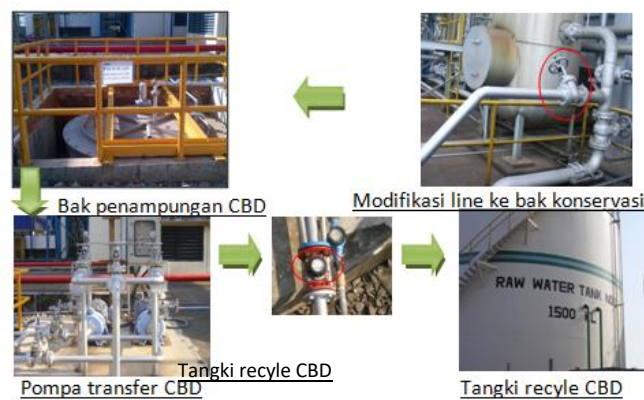
Figure 3. Modification of CBD Water Recycle.
